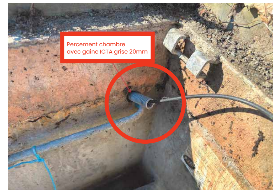
Exemple de percement non standard.
